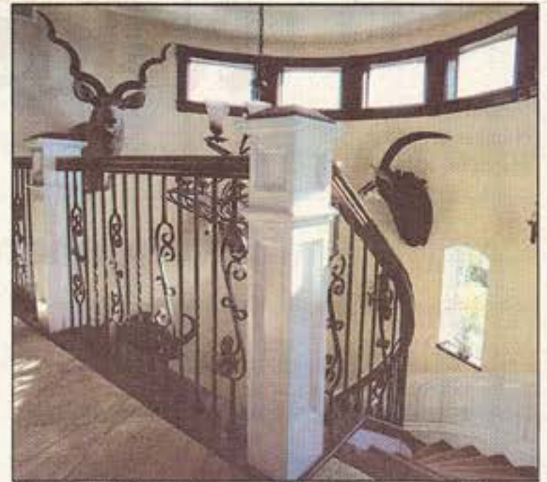
The stairs include extensive upgraded details, such as an oversized curved railing, oversized paneled newels, wrought iron balusters, and custom raised panel wainscot.
